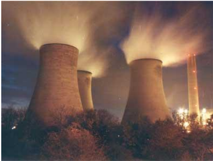
Coal-fired power station ~ 30-35% efficiency
